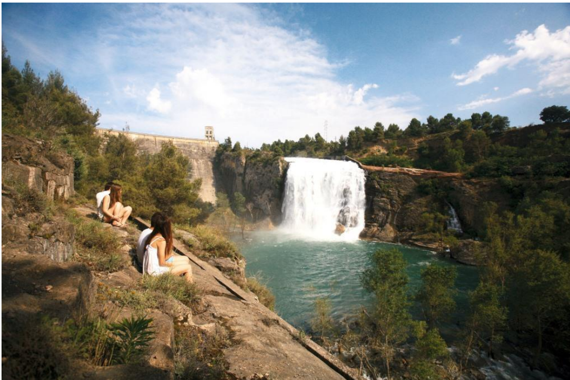
Dam of Talarn
